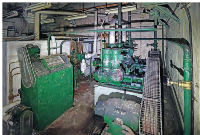
The air conditioning plant room – one of the few rooms that always had a solid floor. It was entered by steps down from the spine corridor
